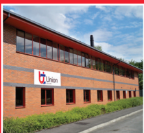
UK Headquarters and Technical Centre
